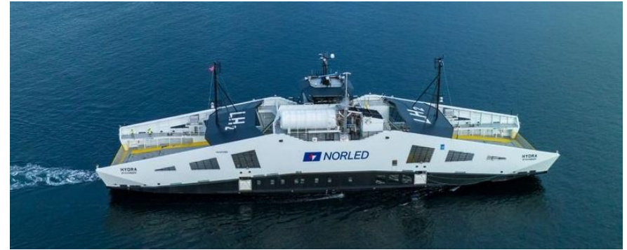
Hydra hydrogen powered ferry, Norway
